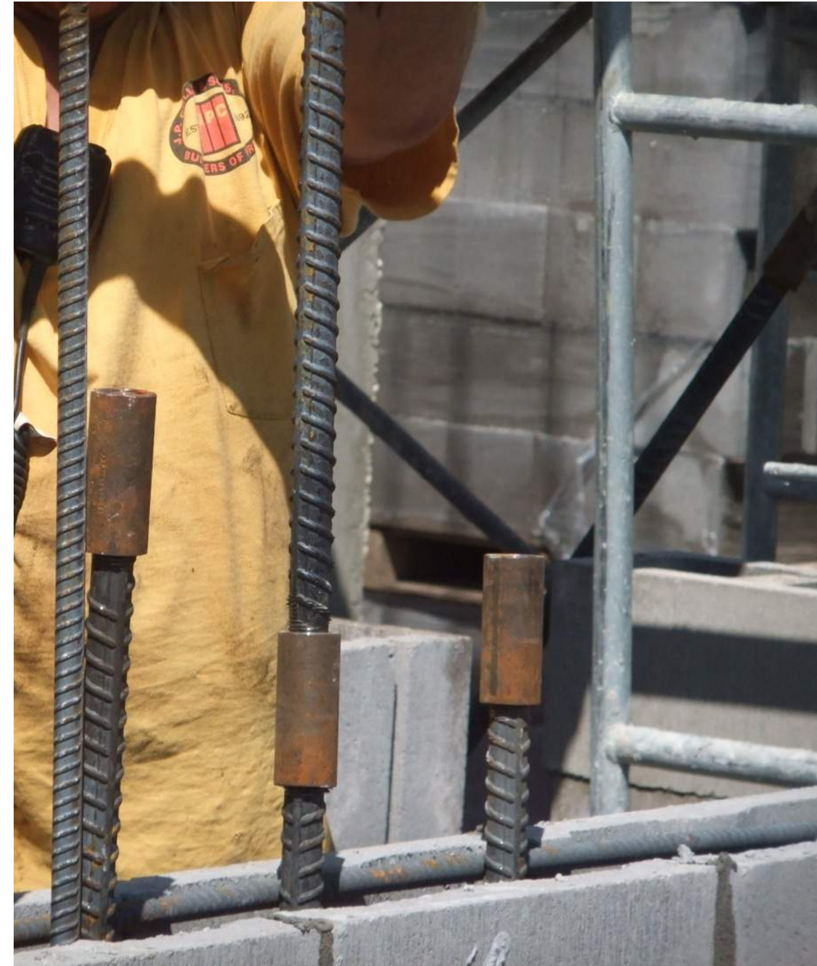
couplers w/ threaded 5'-0" rebar
