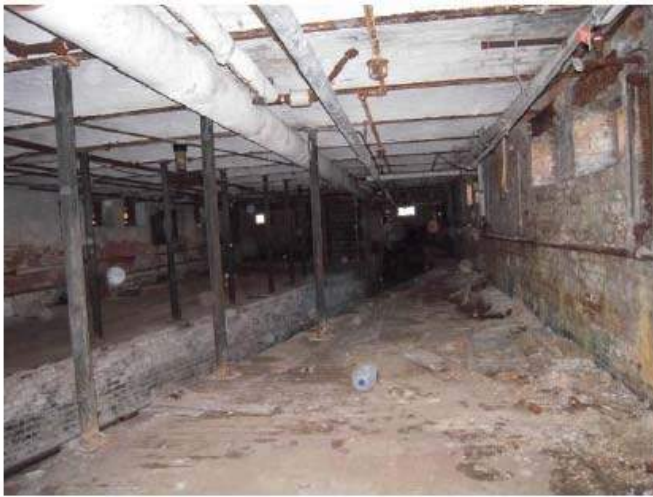
Fig. 38. Brick Floor-arch
