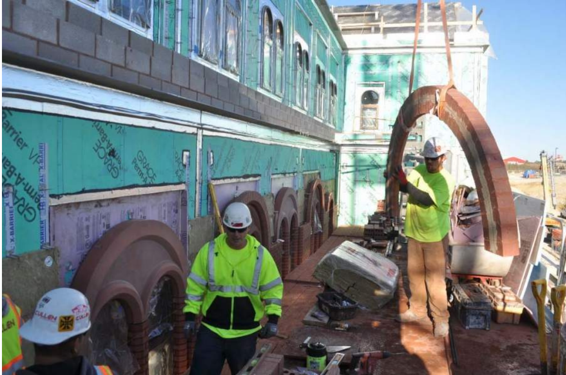
prefabricated masonry arches
