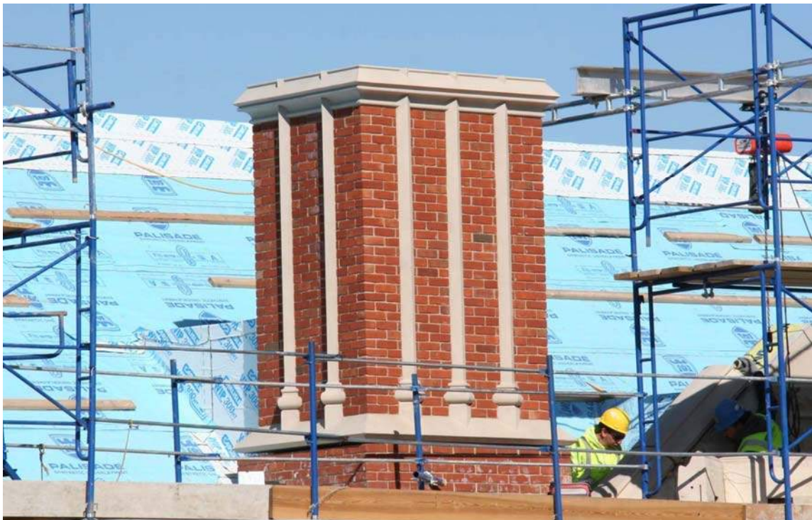
prefabricated masonry chimney
