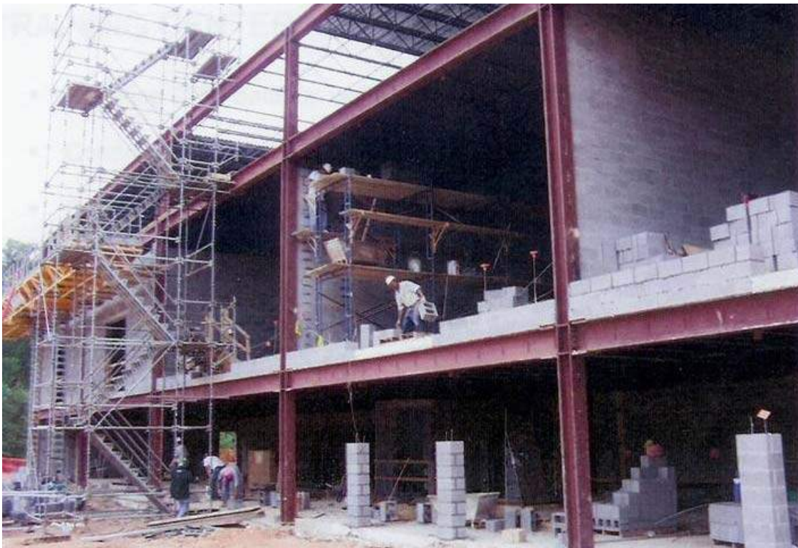
“hybrid” masonry wall w/ steel frame
