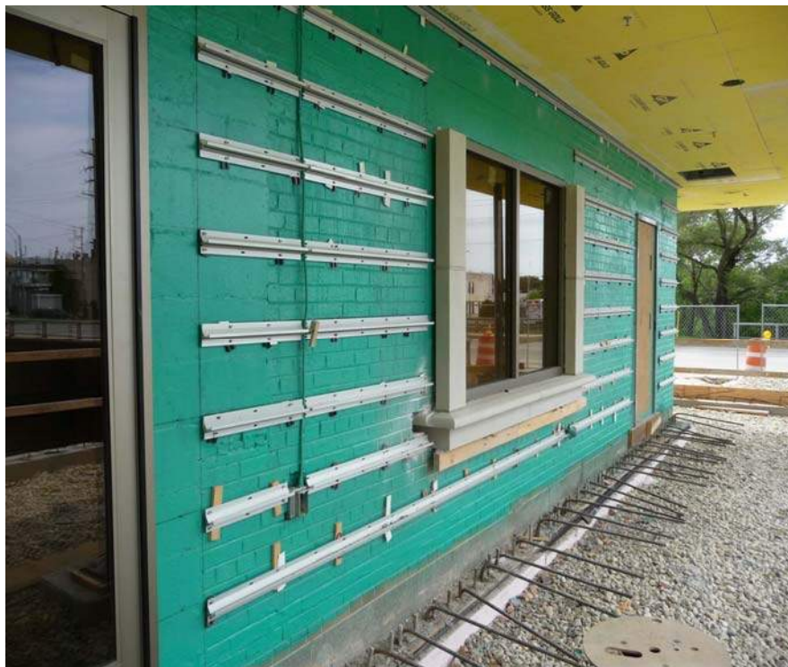
re-clad of existing building
