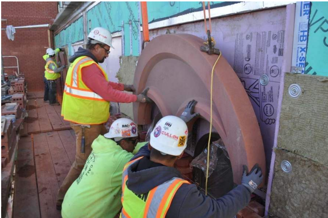
prefabricated masonry arches
