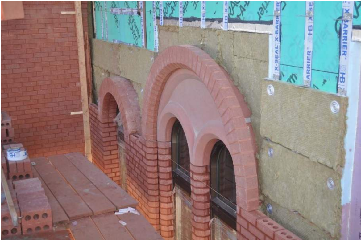
prefabricated masonry arches
