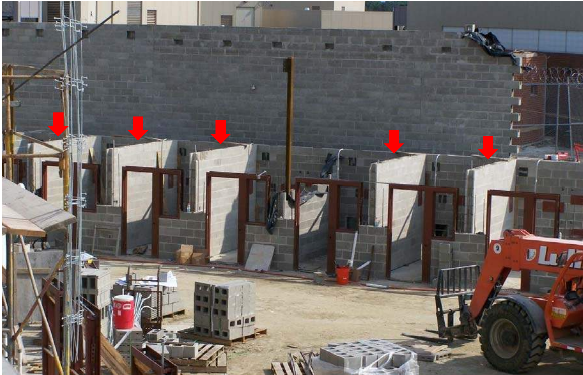
prefabricated CMU panels
