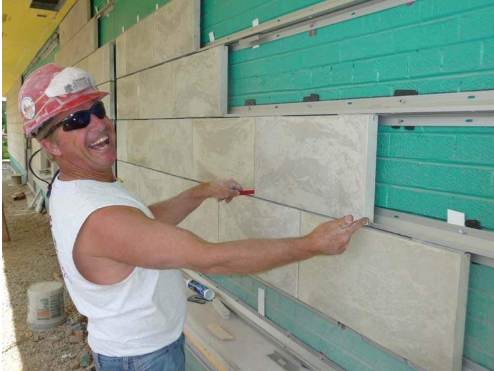
channel-anchored masonry recladding
